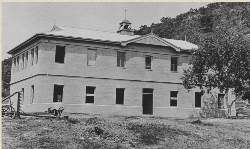
Photos: European Hospital Port Moresby under construction in 1932.
